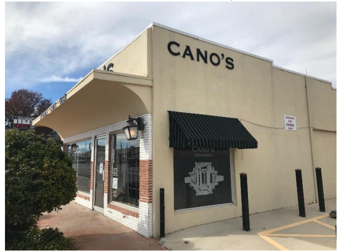
EXAMPLE OF SIMILAR LIGHT FIXTURES (CANO'S 1016 W. BEAUREGARD AVE)
