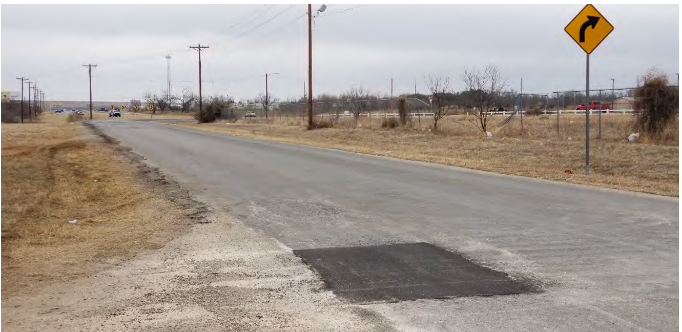
At golf course entrance site looking north to Bryant Blvd. connection
