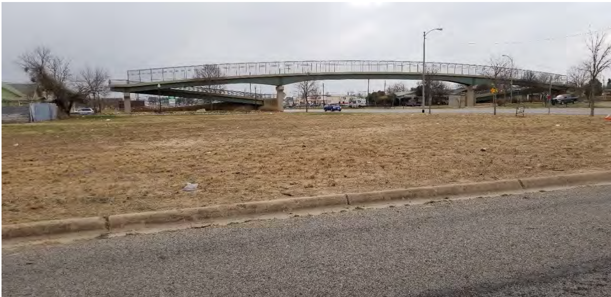
Elevated crossover of S. Bryant Blvd. one block south of CU20-03 site where commercial begins
