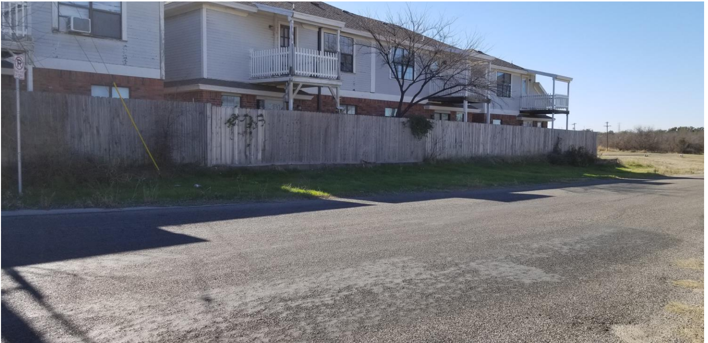
Rear yard of existing townhomes
