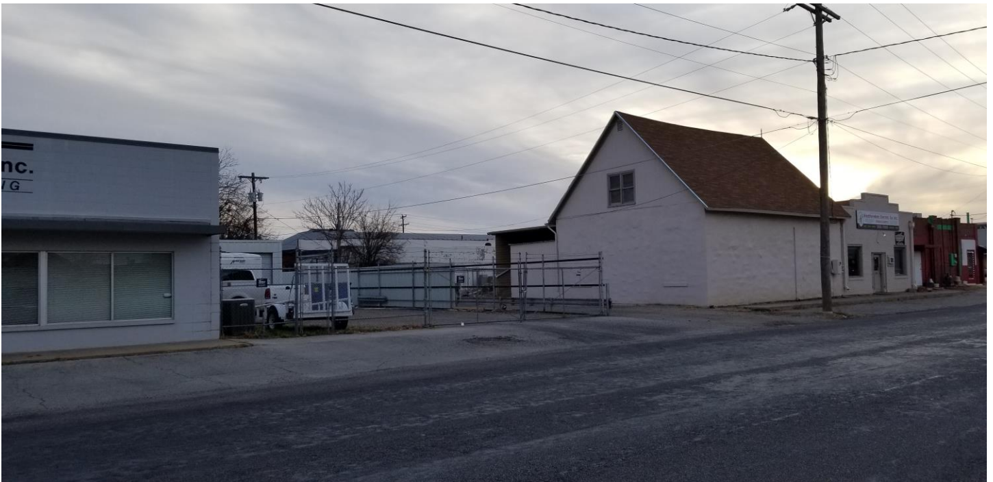
Fence to be replaced with solid 8 ft. metal fence
