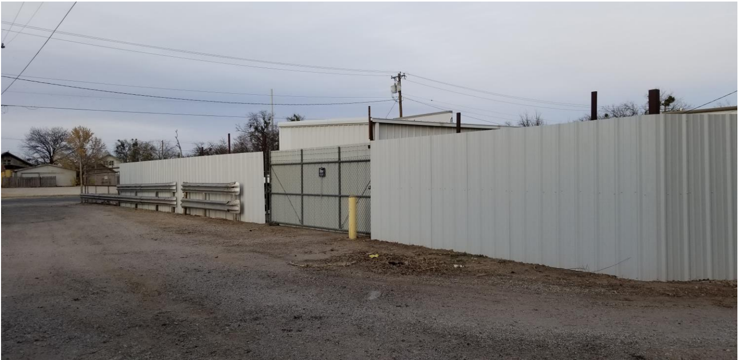
Existing fence in alley to the 25 ft. setback line
