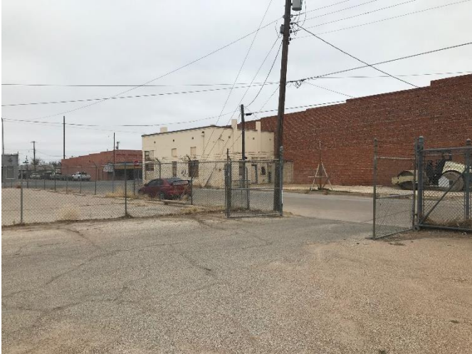
EXISTING PARKING AREA BEHIND BUILDING
