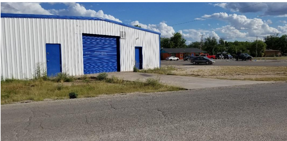
E. 40 th Street paved driveway
