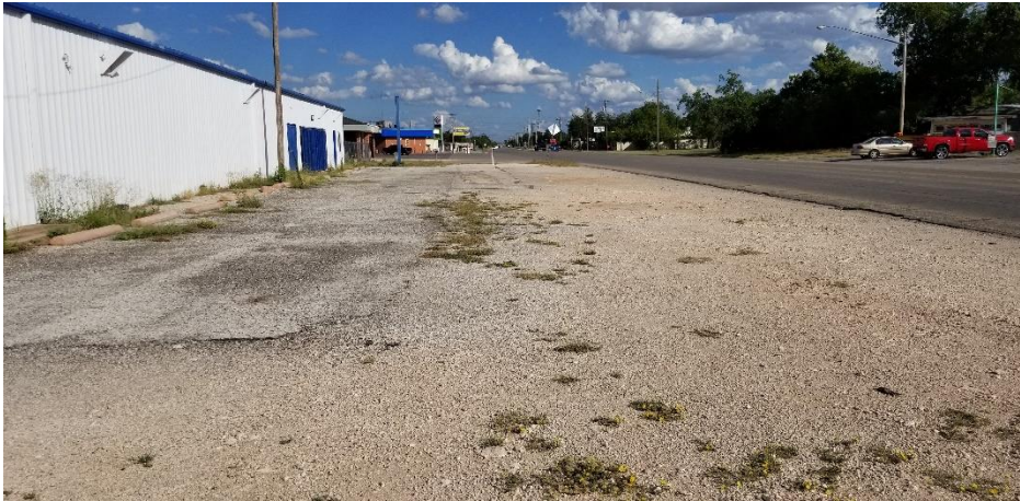
Blue door is tenant space entrance
