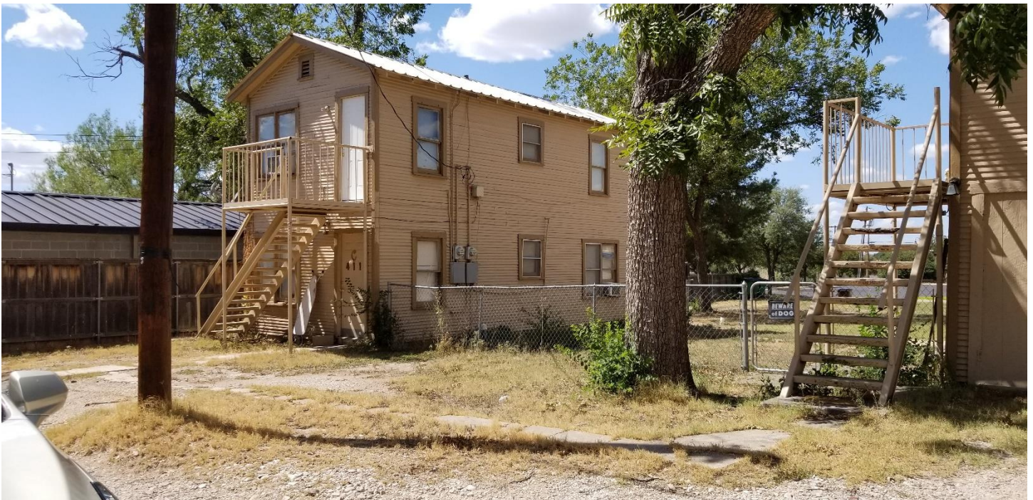
Off the alley – one of the existing two story units
