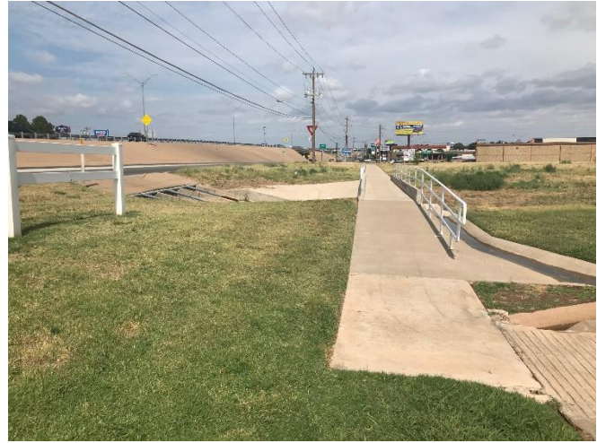
WEST ADJACENT TO LOOP 306
