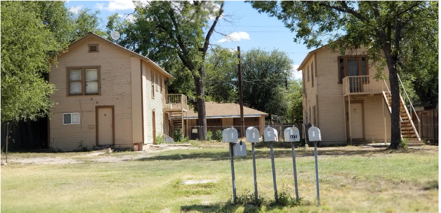
Looking south where the existing two story units.
