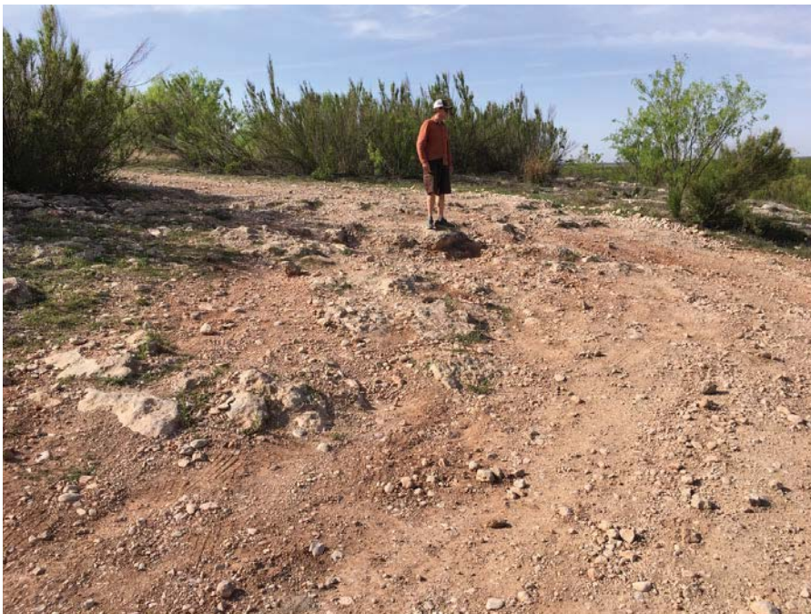
Steep route depositing material directly into reservoir
