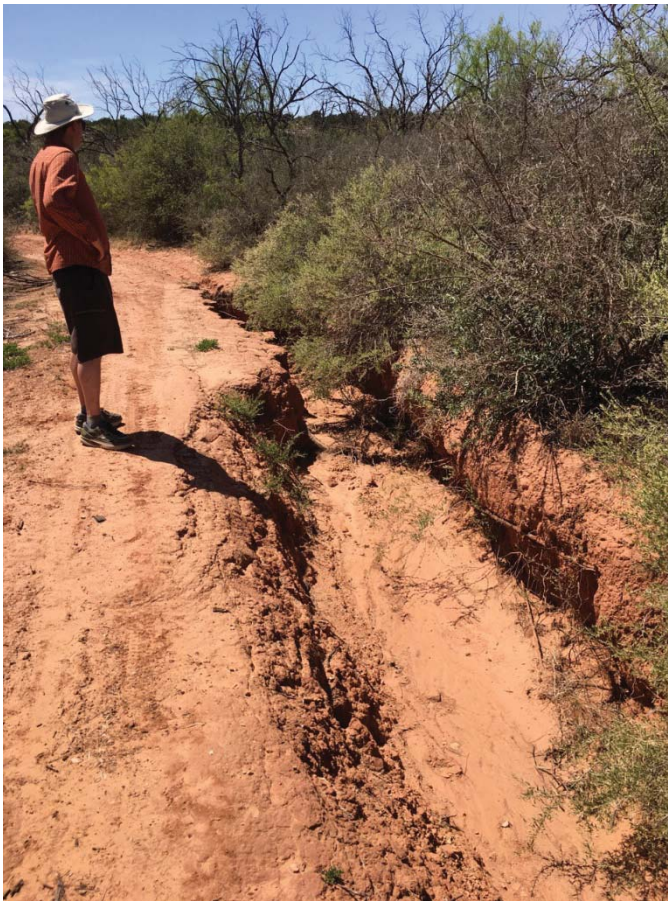
Ruts and rills can lead to an incised route
