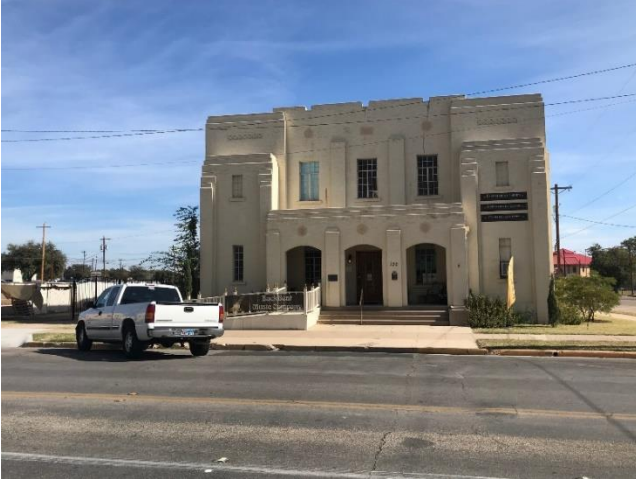
FRONT OF BUILDING
