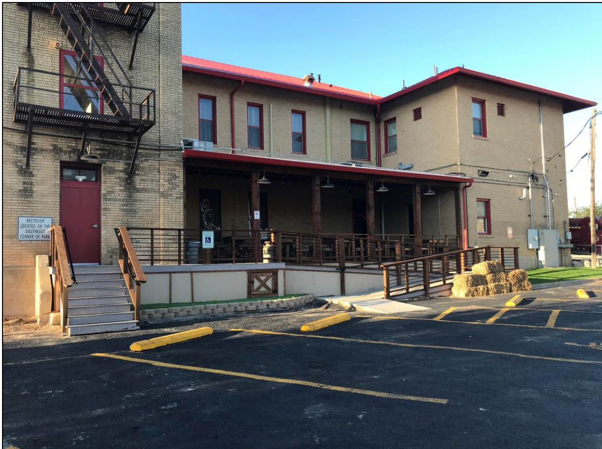
Side of the building
