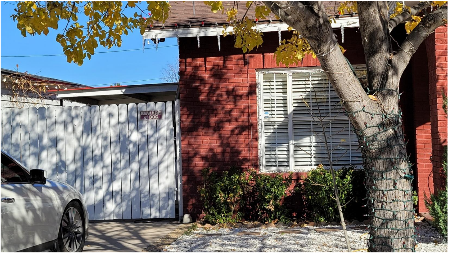
Showing the lending of the carport and roof with the existing home.
