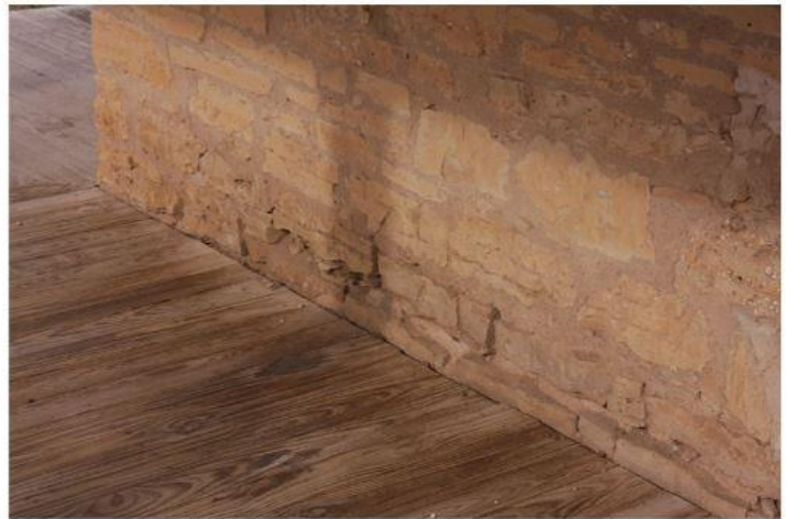
AN EXCELLANT EXAMPLE OF STONE COLOR AND SMALLER STONE PATTERN USED WHICH WOULD HAVE BEEN USED BY THE BUFFALO SOLDIERS WHEN CONSTRUCTING BARRACKS 3 AND 4
