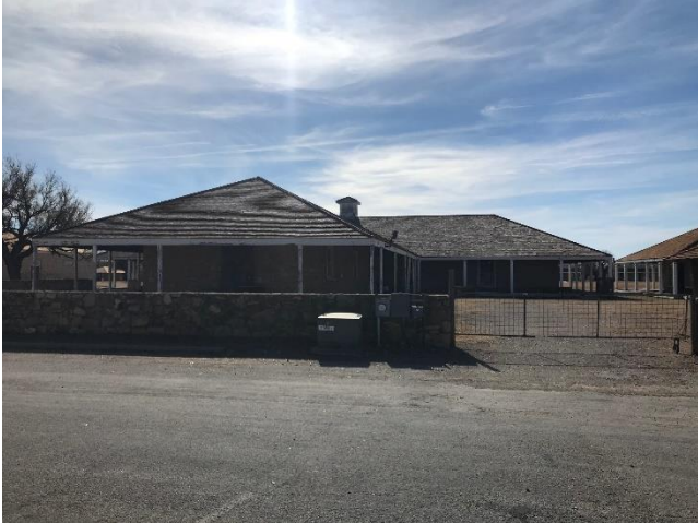
BMH6 LOOKING SOUTH
