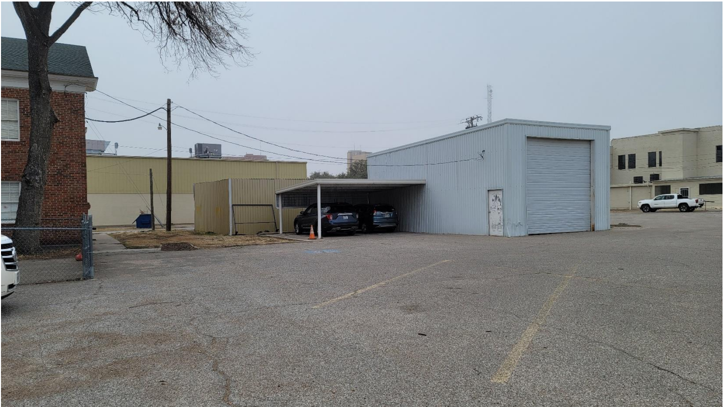
Metal buildings to be removed for reconfiguration of parking lot and playground placement next to church.
