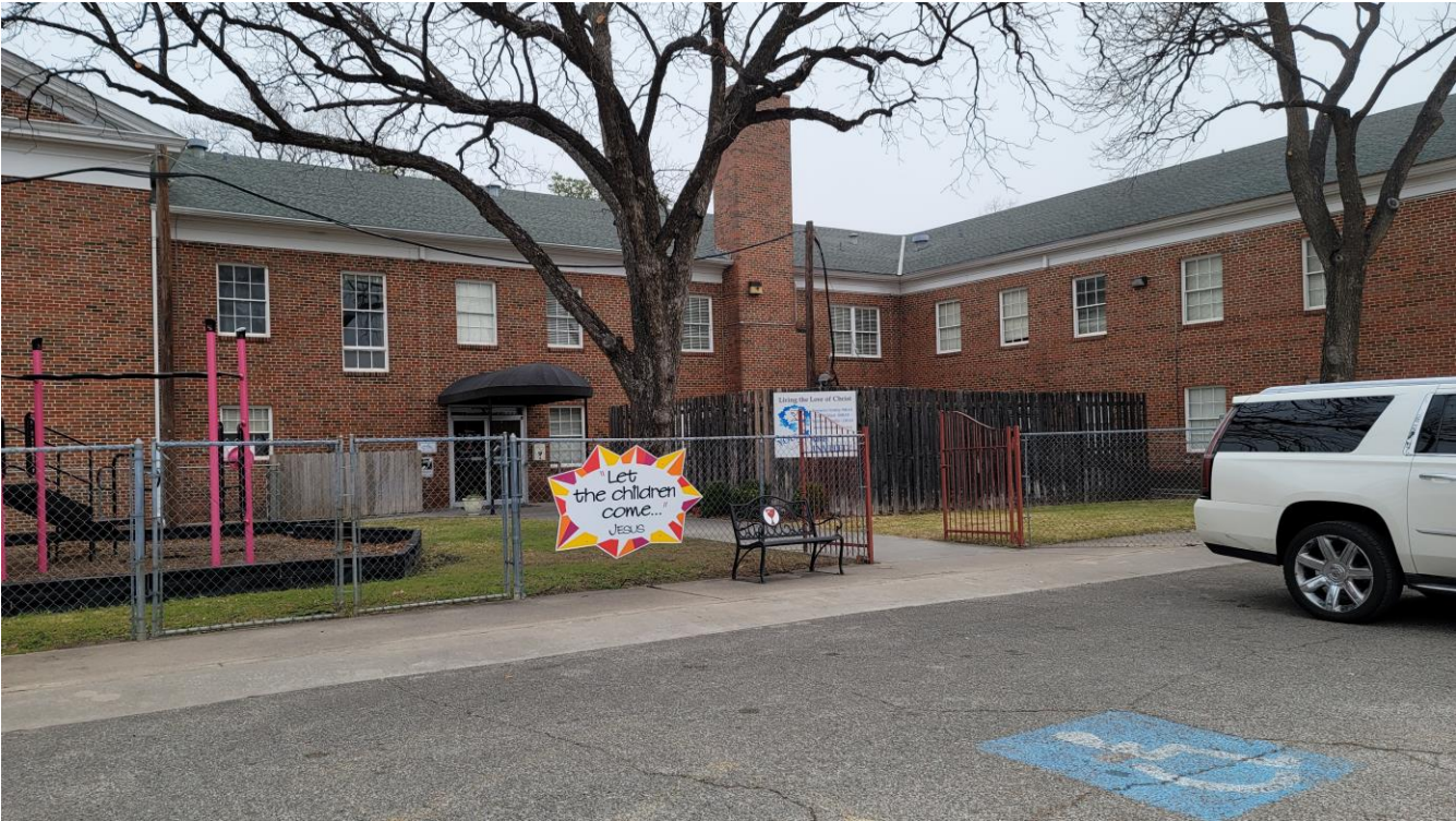
Chiller fencing to be replaced, "The Table" sign painted on fence.
