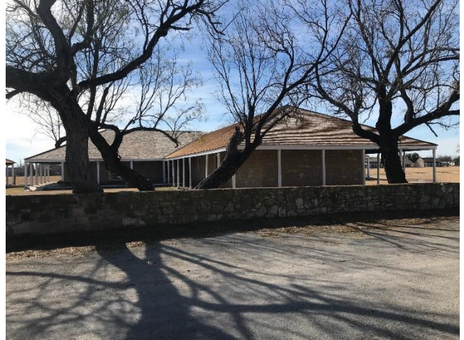
BMH5 LOOKING SOUTH
