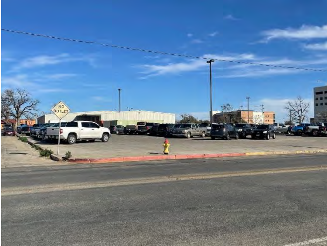
EXISTING MAINTENANCE FACILITY (WOODROW ST)
