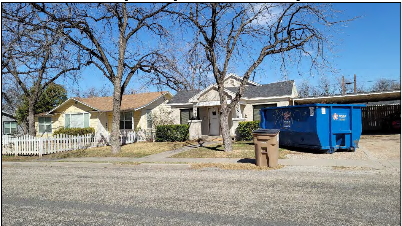
Existing house being remodeled for household living.
