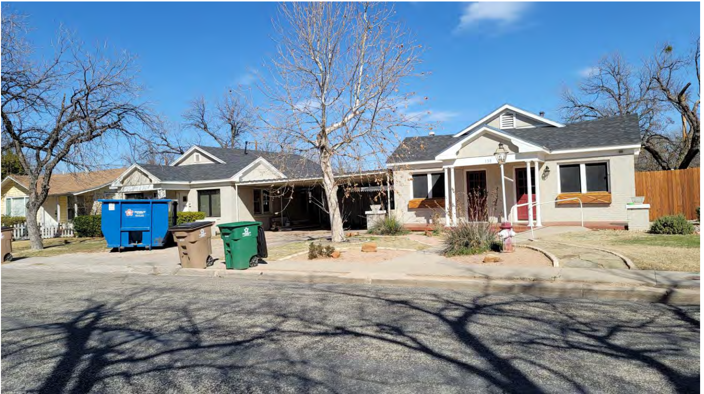
Existing office that will remain. Next door to Conditional Use structure.
