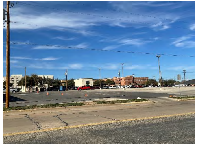
TWOHIG AVE. – FUTURE PARKING GARAGE
