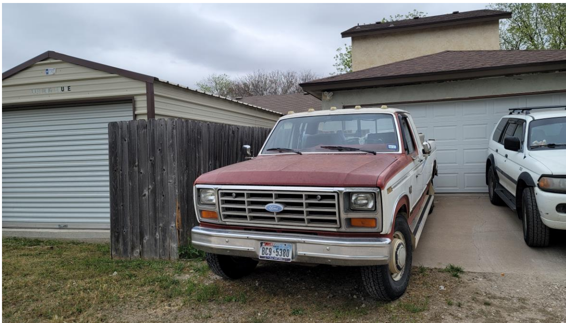
Picture shows the closeness of the house/garage structure and the neighbor's garage.
