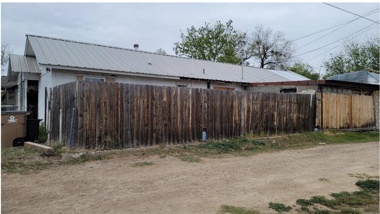
Front of house with fencing covering the enclosed carport.
