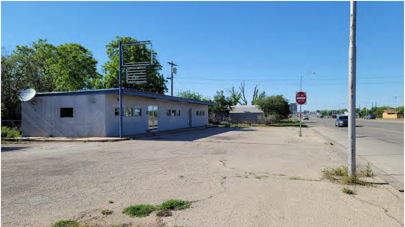
2321 South Bryant Blvd. existing access curb cut off Bryant.
