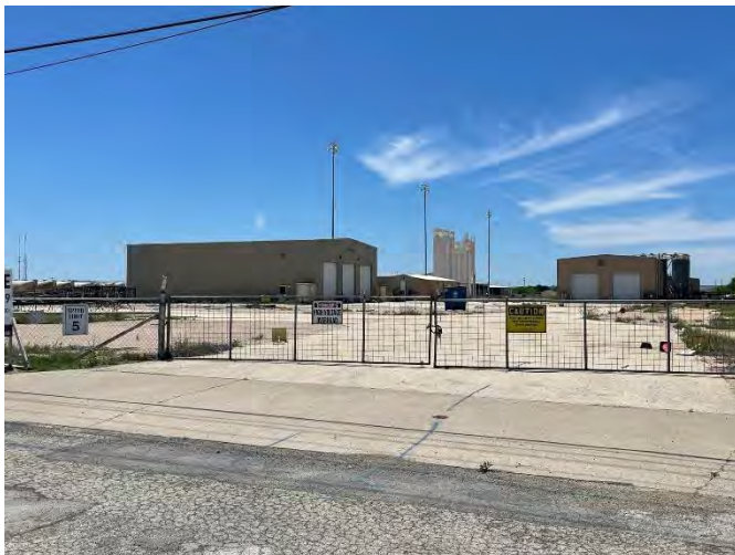
NORTHWEST AT SUBJECT PROPERTY
