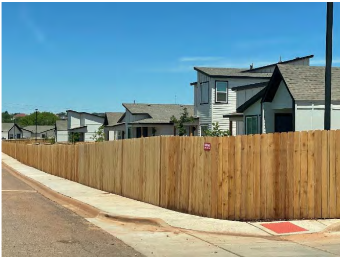
MIDDLE VIEW OF FRONT FENCE
