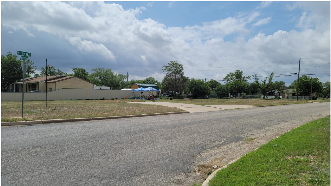
View of the variance Irene Street side with curb and gutter.
