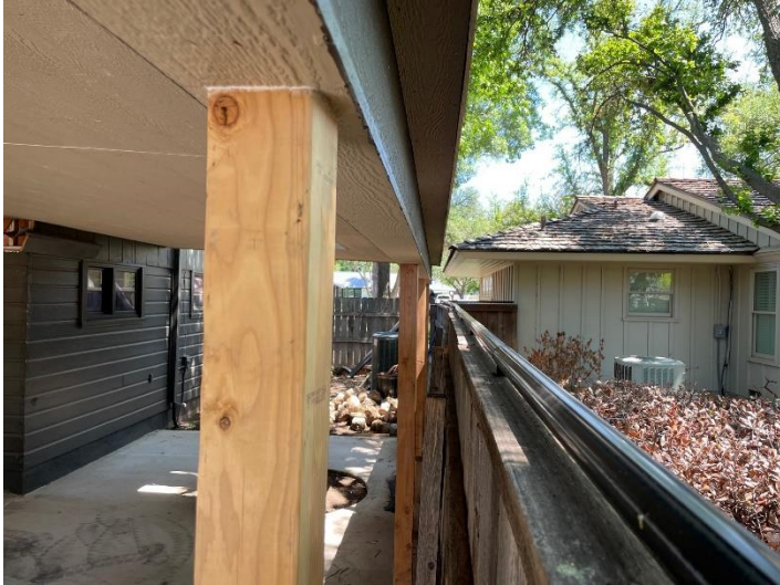
LOOKING NORTH AT WEST SIDE
