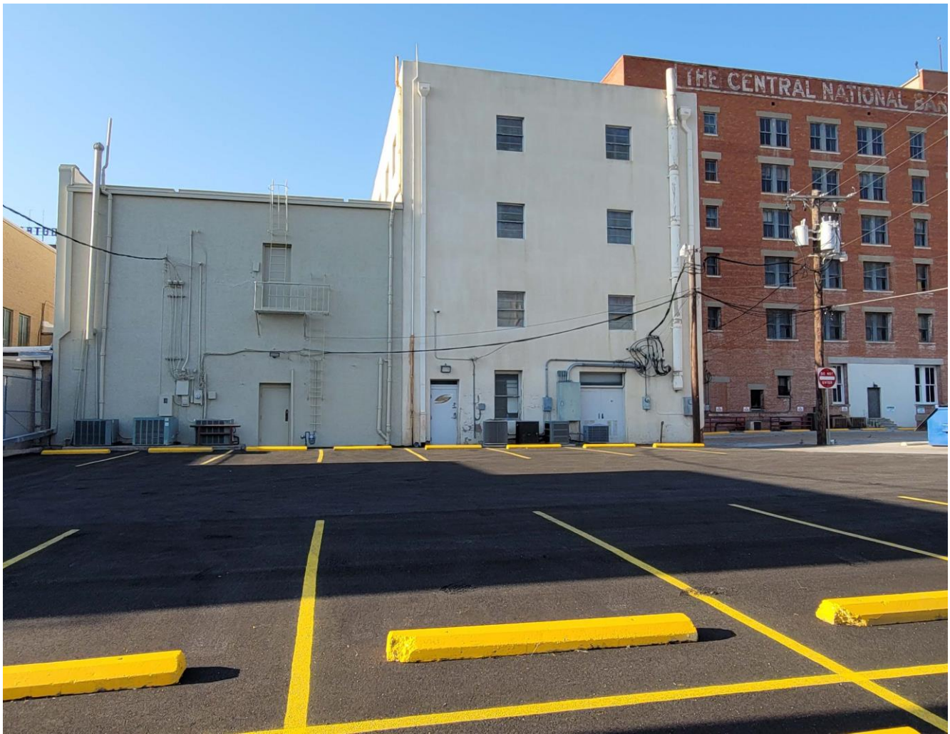
Changes to the back of 16 East Beauregard including painting, refurbished parking area and striping.
