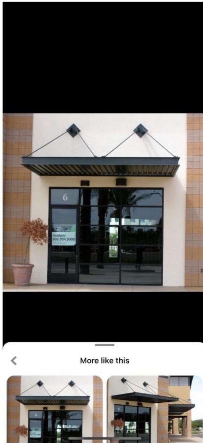
Shows an example of intended awning and placement over window array. 9 ft. 1 inch from sidewalk to bottom of awning. Awning is powder coated matte black metal, about a foot from window and door to awning bottom.
