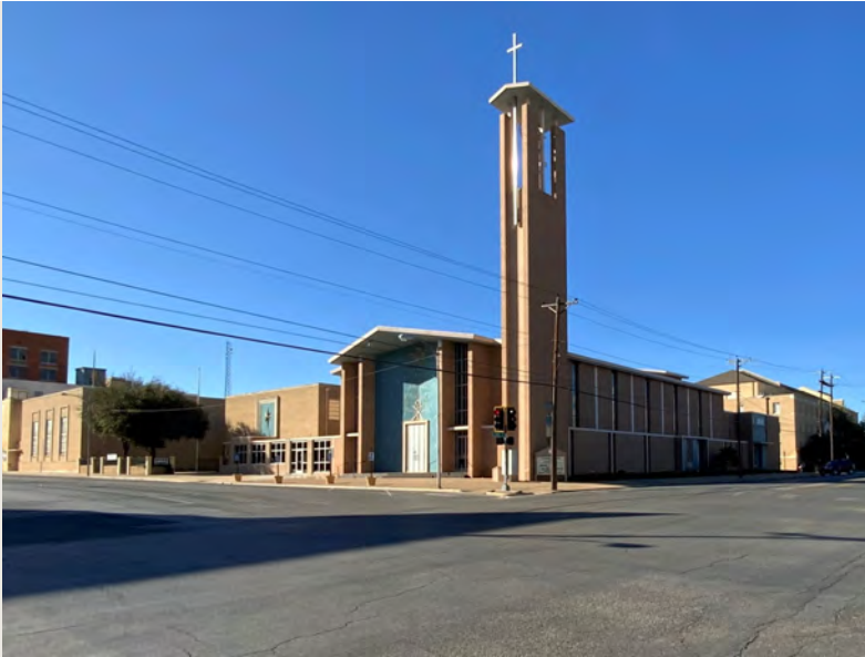
Figure 2-26. Sacred Heart Catholic Church, 19 S. Oakes Street, designed by Henry Steinbomber, constructed by Templeton and Cannon (1960-1961). Photo by HHM, 2020.
