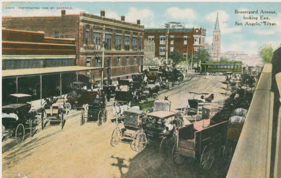
Figure 2-17. Postcard of a typical commercial streetscape, 1911, along Beaugard Avenue. Source: M.C. Ragsdale [Beaugard Avenue in San Angelo], postcard, September 1911, from the Portal to Texas History, crediting Permian Basin Petroleum Museum, Library and Hall of Fame, https://texashistory.unt.edu/ark:/67531/metaph1129223 .
