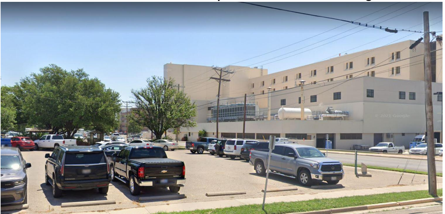
Shannon Medical Center West Expansion- viewed from College Ave.
