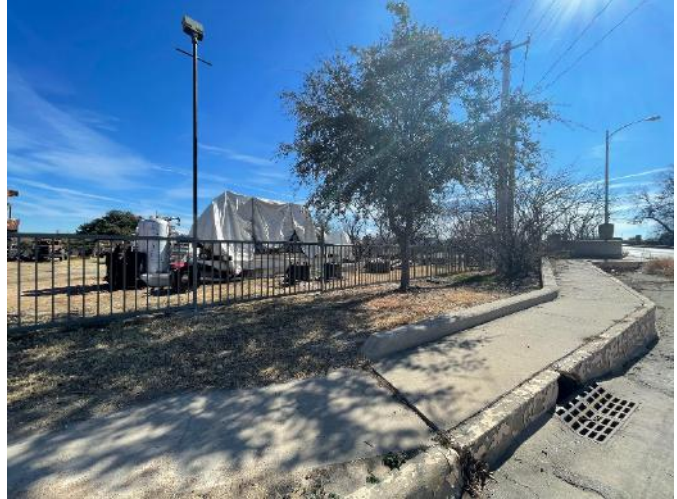
SOUTHEAST AT PROPERTY
