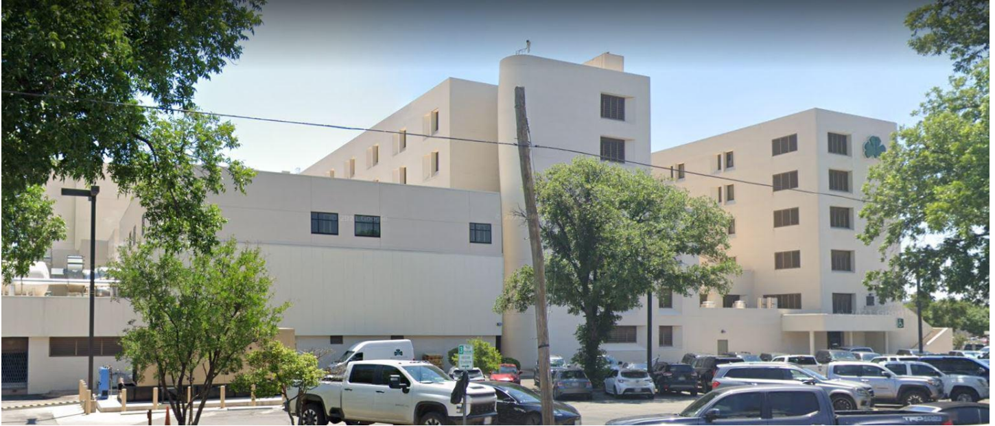
Shannon Medical Center West Expansion- viewed from N. Oakes St.
