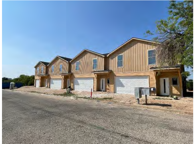
NEW TOWNHOMES UNDER CONSTRUCTION (1012-1024 HOLIDAY DRIVE)
