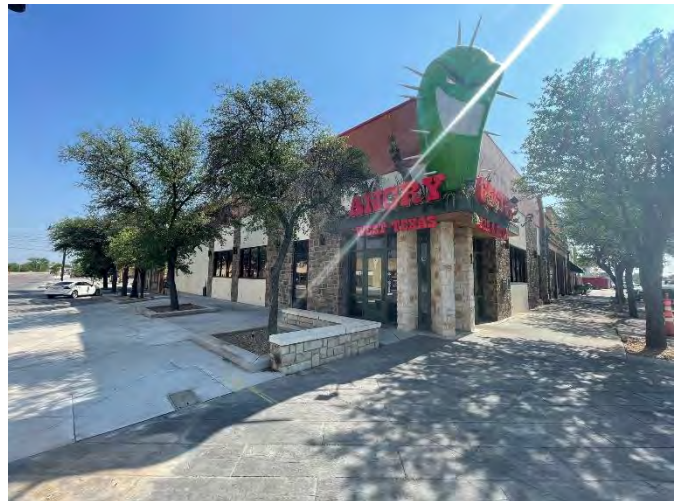
CORNER VIEW OF 1 W. CONCHO AVENUE
