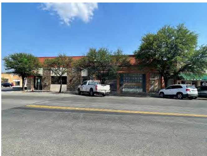
LOOKING SOUTH AT 1 AND 5 W. CONCHO AVENUE
