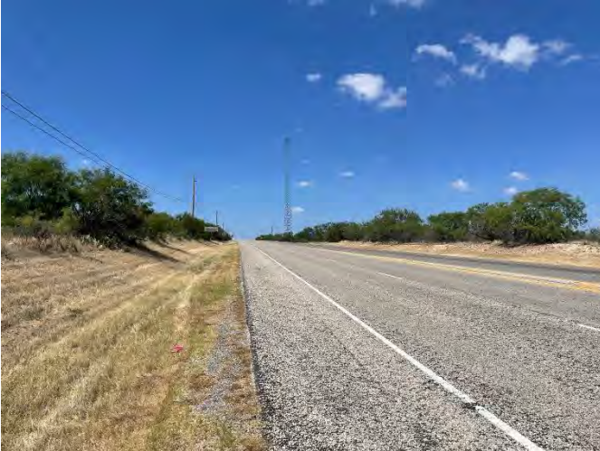
NORTHBOUND ON ARDEN RD.
