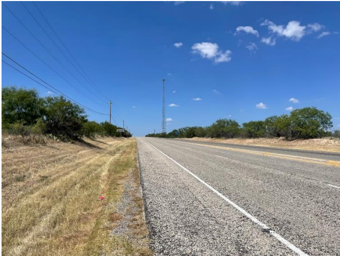
NORTHBOUND ON ARDEN RD.
