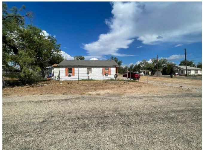
EAST AT PROPERTY ACROSS STREET
