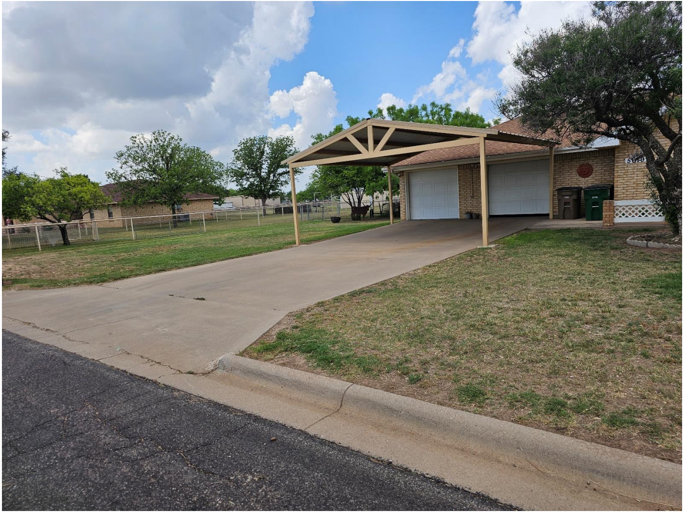
The detail on the carport shows the matching color scheme, the matching roof pitch, and the construction attempt to blend with the home.
