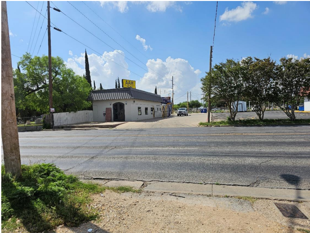
OVERALL PICTURE OF THE SITE SHOWING NEIGHBORHOOD
