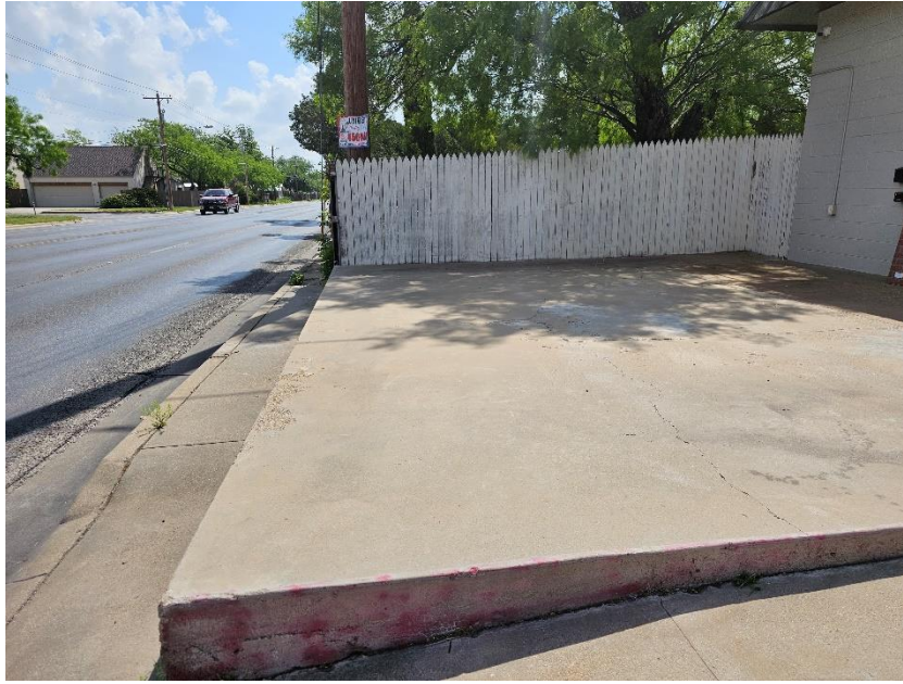
EXISTING CONCRETE PAD SHOWING IT IS ADJACENT TO SIDEWALK
