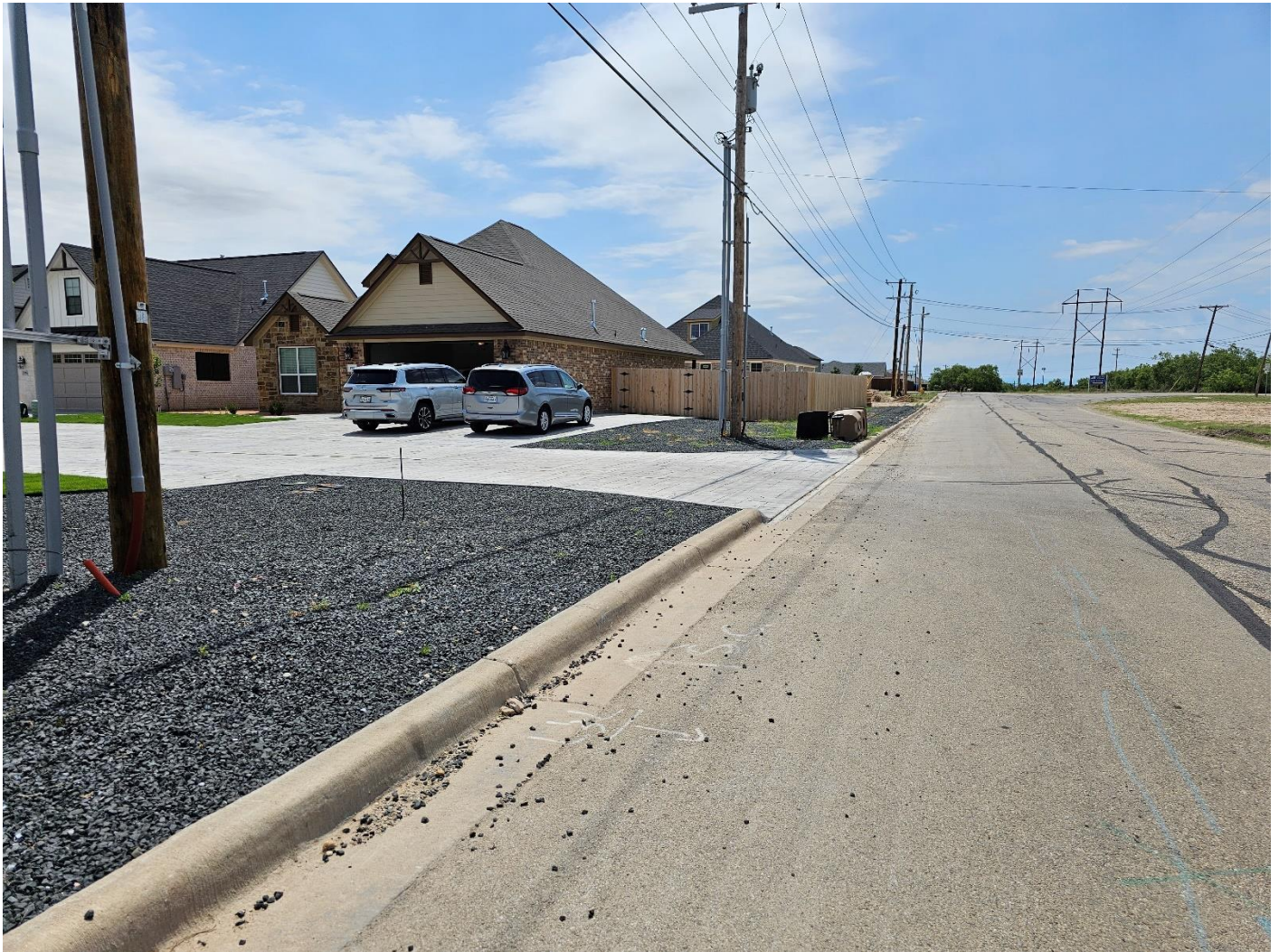
View showing a 15-foot street side front yard setback
