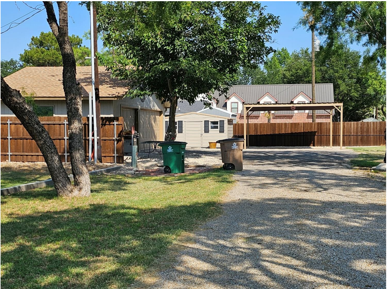
Adjacent home accessory structure and carport built in the easement.
