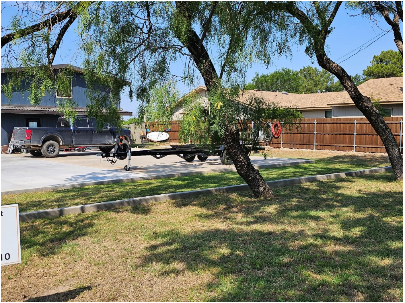
The applicant's property shows the concrete slab on which he intends to build the attached garage. From the slab to the concrete property marker is 11 feet.
