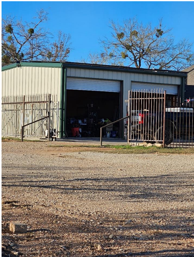
Shows fence requiring variance as well as shop.
