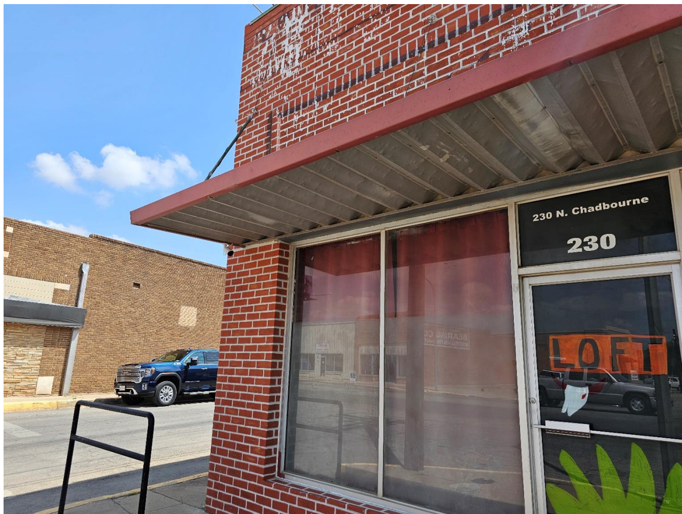
Showing the stucco wall to be removed and the glass to be replaced.
