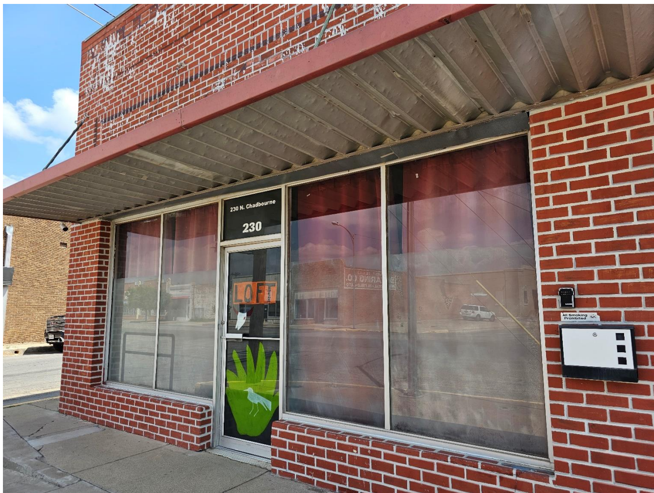
Showing the awning to be refurbished and repainted.
