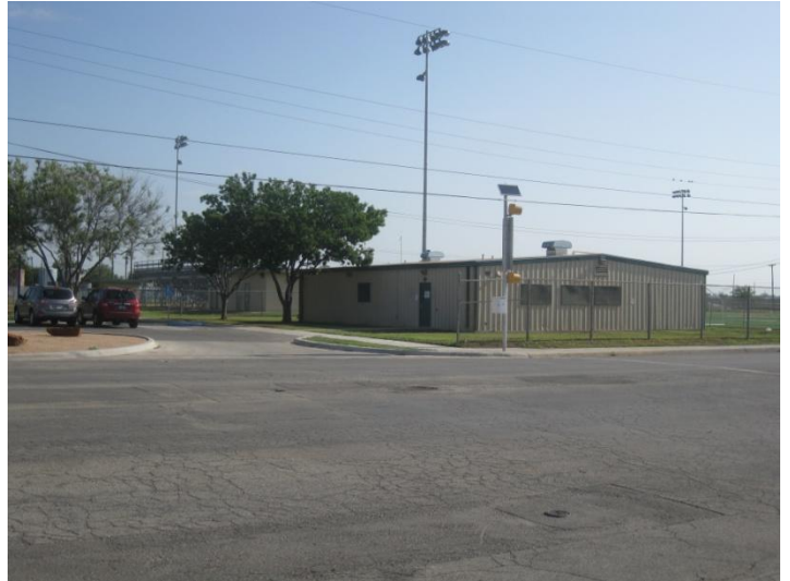
Looking north – east part of property (Portable building – future sign location)
