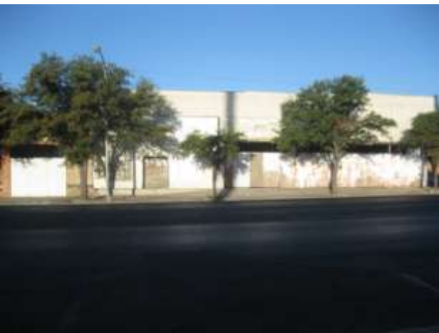
Looking East at building (S. Chadbourne)
