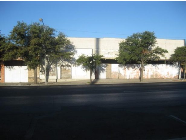
Looking East at building (S. Chadbourne)
