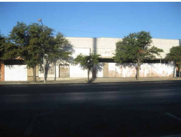
Looking East at building (S. Chadbourne)
