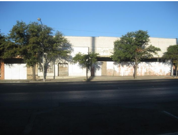
Looking East at building (S. Chadbourne)
